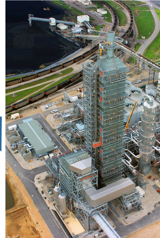
Petra Nova, world's largest post-combustion CO 2 capture plant, began operation in January 2017 (240 MW)
